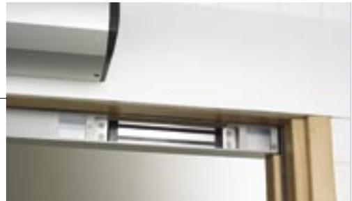
The Dor-O-Matic unit is linked to an electromagnetic lock surface mounted to the underside of the frame, with the armature mounted on the door face. When the door is activated from inside, it initiates the system to 'close and lock' or 'unlock and open'.
