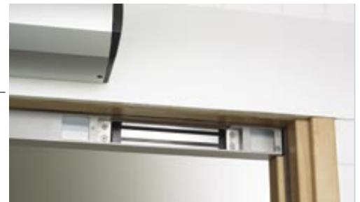
The Dor-O-Matic unit is linked to an electromagnetic lock, surface mounted to the underside of the frame, with the armature mounted on the door face. When the activation pad is pressed from inside, it initiates the system to *close and lock* or *unlock and open*.
